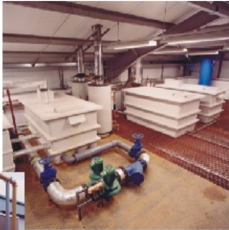
Hatchery chiller (left) and water storage tanks
